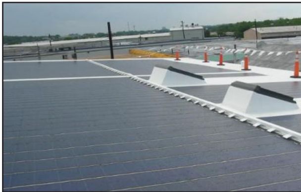
The James Myers Company Beltsville, MD – 14 kW PV System
