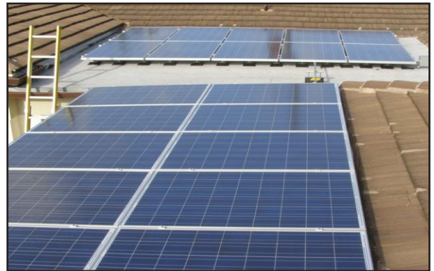
Florida Residence – 4000 Watt PV System
