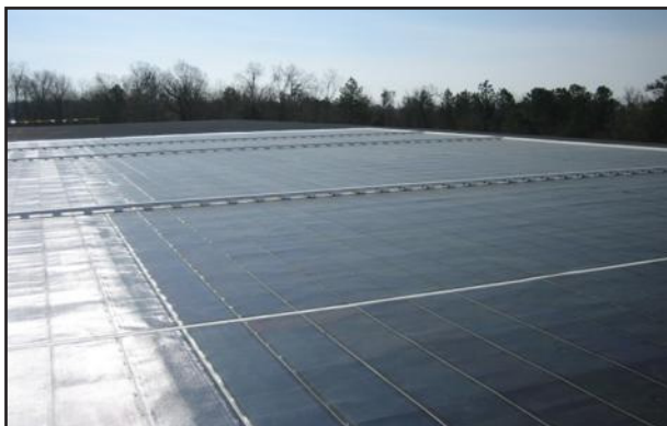
The Hamlin Companies Benon, NC 107 kW – PV System
