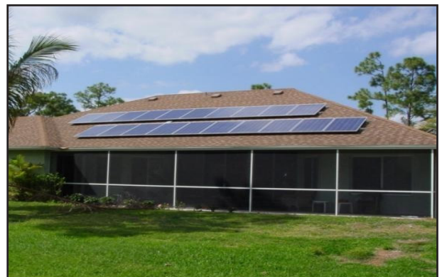
Florida Residence – 4000 Watt PV System
